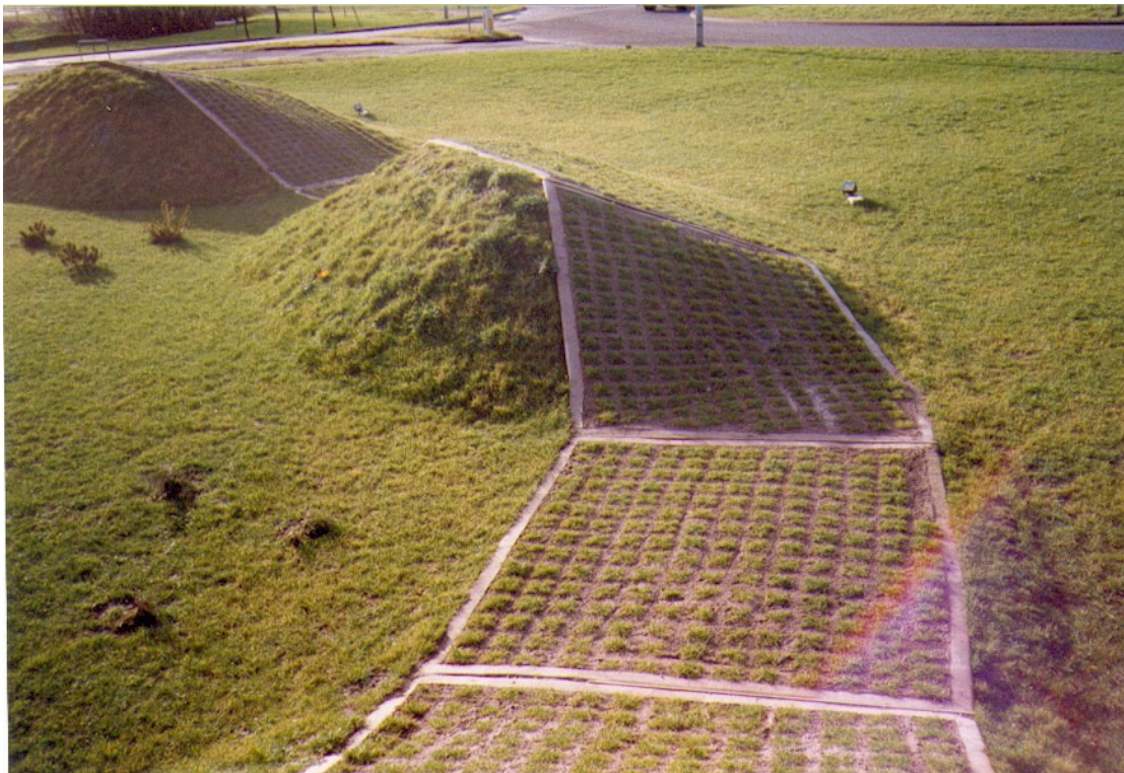
The photograph shows Grasscrete with the solid concrete edges used as essential delineation for safe passage
